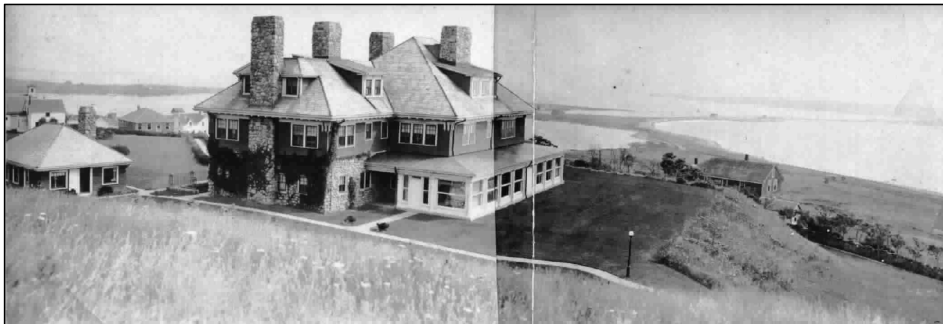
The growth of ivy over the stone façade and chimney and the barren landscape probably date this photograph in the early to mid 1930s. CHS collection.
