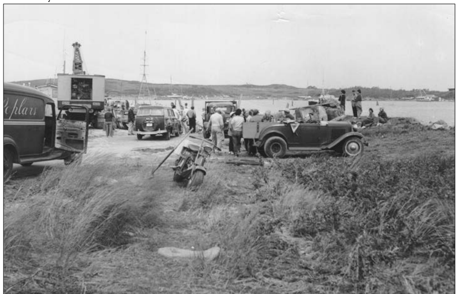
Islanders gather to inspect the damage at the Main Dock.
