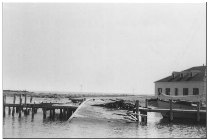
The Coast Guard boathouse survived, but the Main Dock suffered serious damage.
