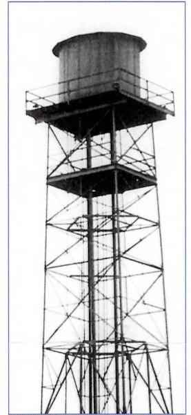
Radar Tower on Cuttyhunk's southwest bluff.
