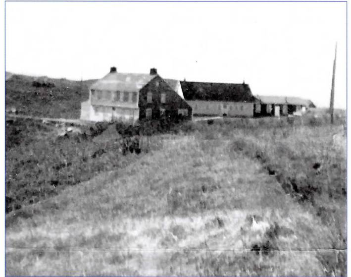
The Central Barracks on Cuttyhunk, showing (from left to right) barracks, mess hall, and annex, circa 1943.
